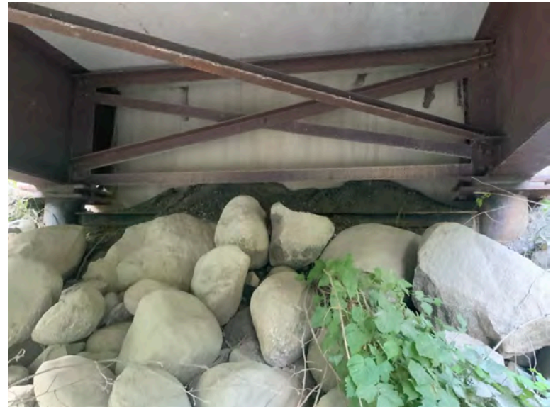
Left Bank Abutment when facing downstream
