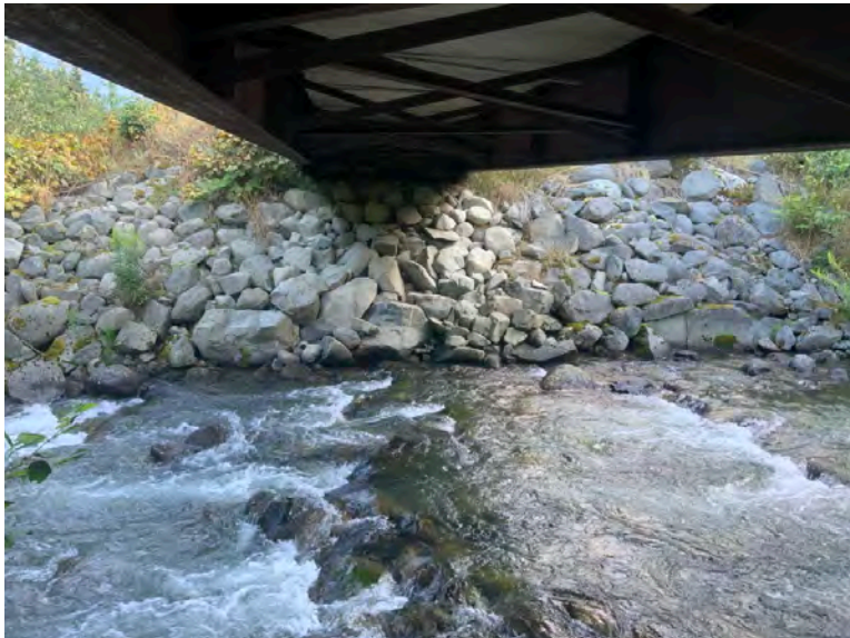
Right Bank Abutment when facing downstream
