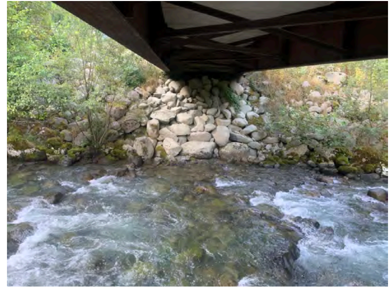
Left Bank Abutment when facing downstream
