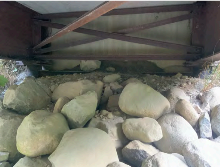
Right Bank Abutment when facing downstream
